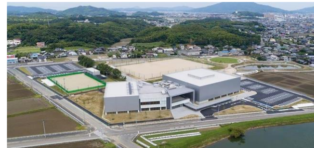
Itoshima City Exercise Park (The front building is a multi-purpose gymnasium)
